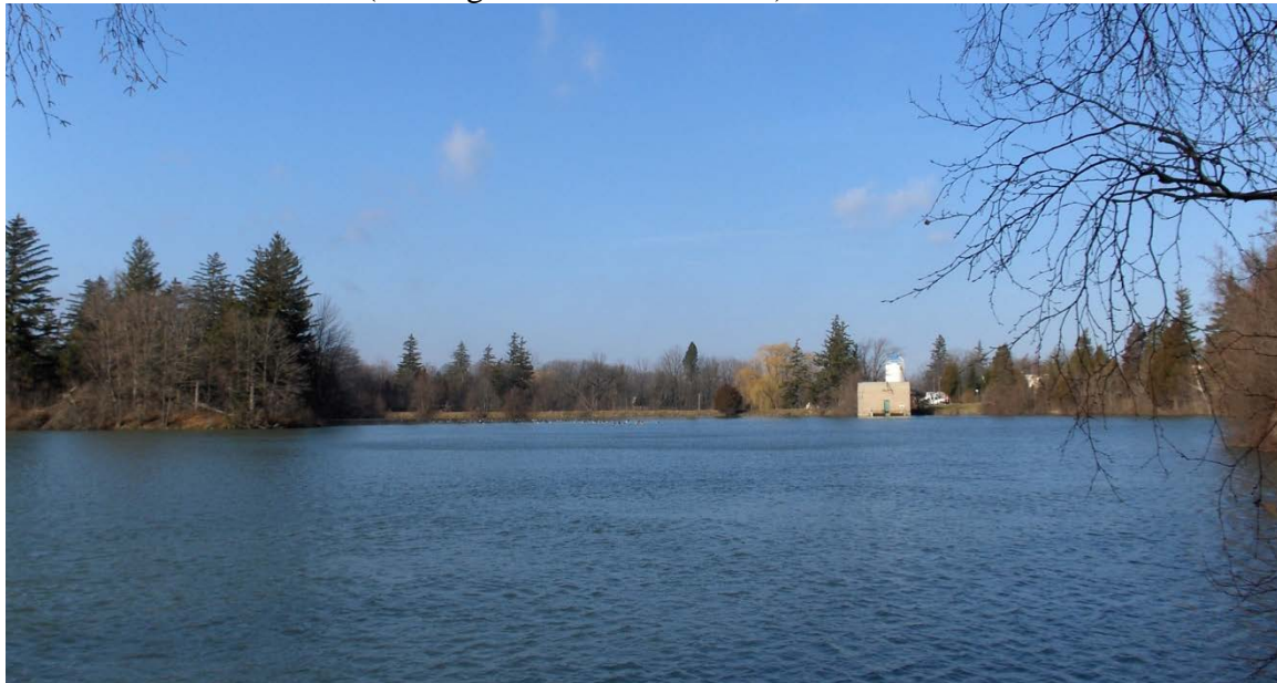
DeCew Lower Reservoir (looking west towards intake)
