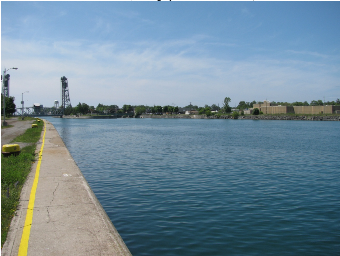
Welland Canal in Port Colborne (looking upstream / to the south)
