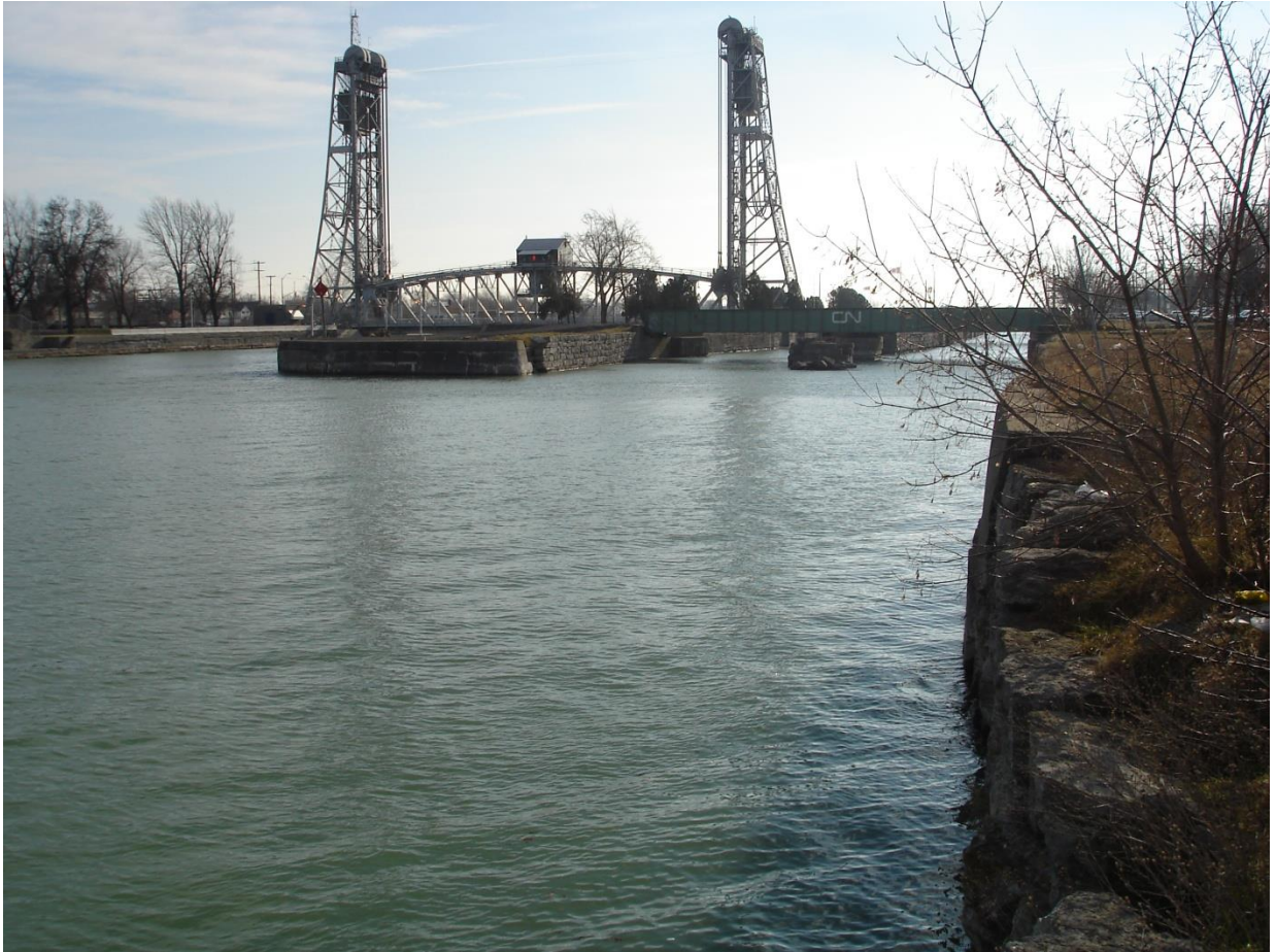
Southerly view from Port Colborne intake
