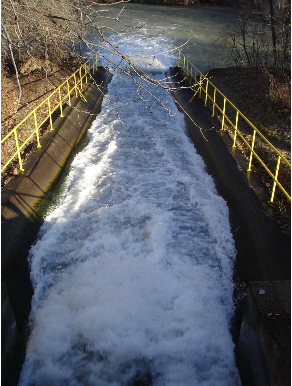
Northerly view from DeCew Supply Weir Tailrace
