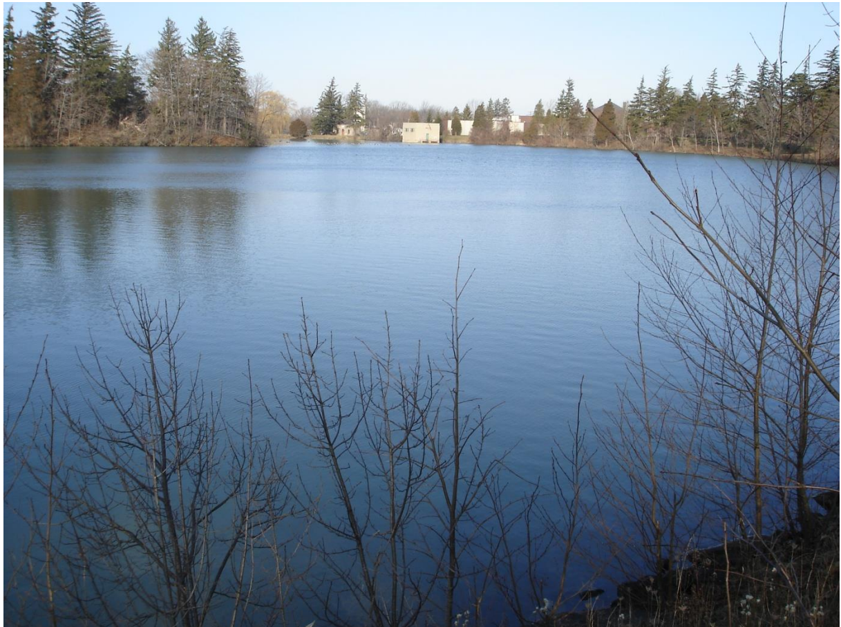
Northwest view of DeCew Main Intake Lower Reservoir
